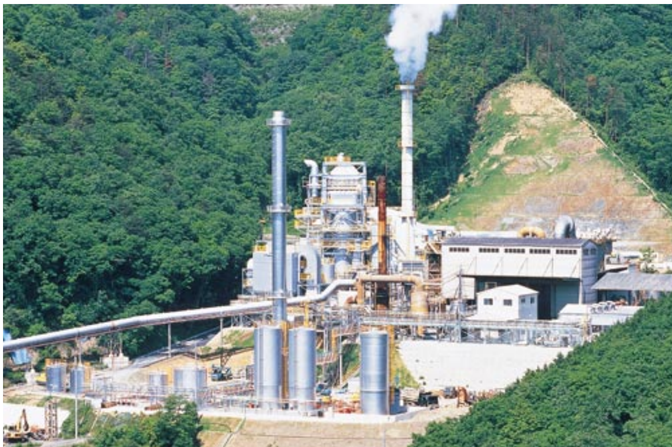
Industrial waste treatment facility
