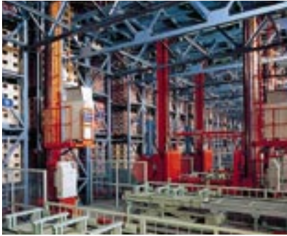
Automated storage and shipping system
