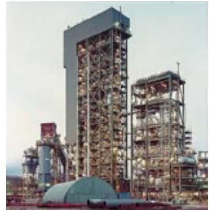
Gasification reactor designed by Krupp Uhde GmbH
