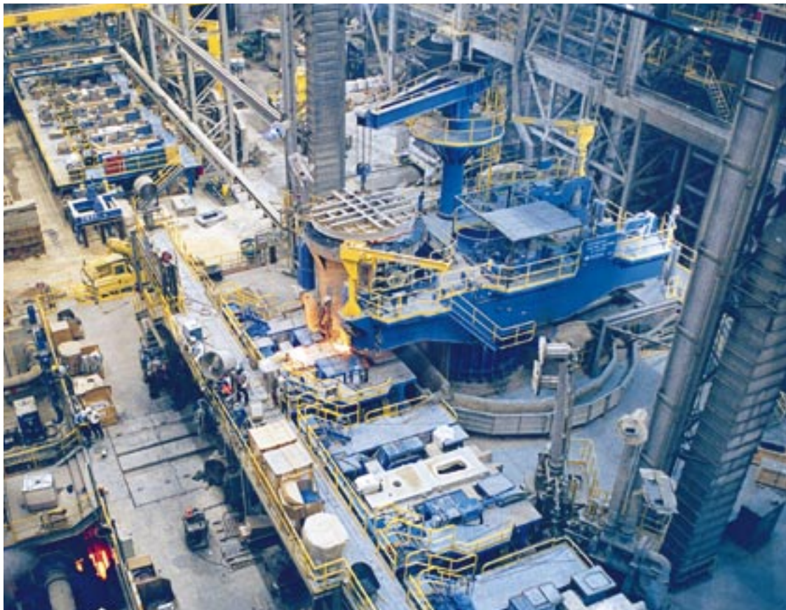
Medium slab continuous casting machine
