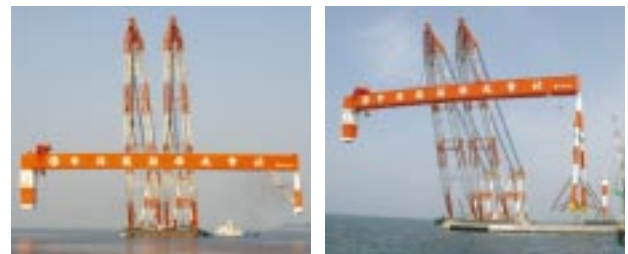
図3 据付け状況 Installation condition
