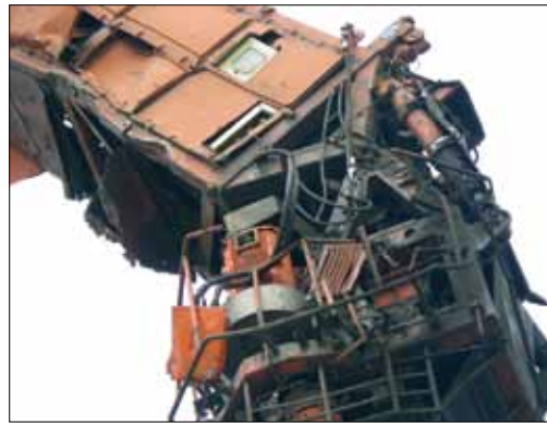
図7 先端掘削部破損 Broken excavator
