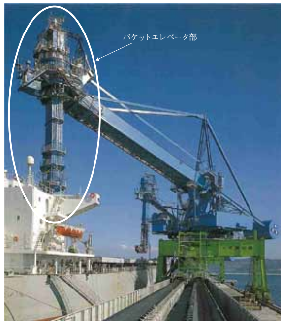
図1 連続式揚炭機外観 Continuous coal unloader
