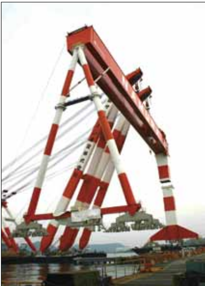
図2 海上組立て Lift of a work by floating crane
